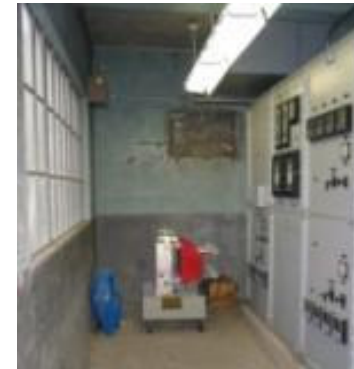
Electric System Upgrades Navy 4 kV to SCL 2.6 kV
