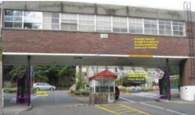
NE 74 th St Intersection Improvements
